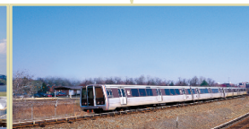
Dulles Corridor Metrorail Project
